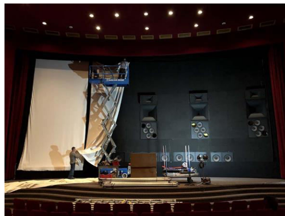
The theater closed in February for the renovation.
